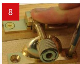
8 While in this position, mark out the screw holes.
