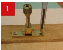
1 When you are happy with the position of the Fastener, making sure the Fastener is in line with the edge of the Sash, mark out the screw holes.
