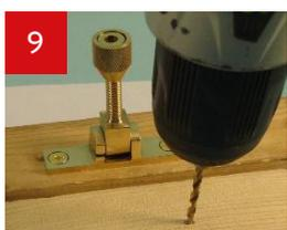
9 Drill out the pilot holes, remove any sawdust.
