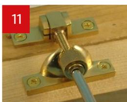
11 Un-tighten the Cap (you will be able to slacken off the Cap without taking it off the Arm of the Fastener so not to lose it).
