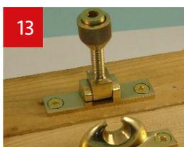
13 The Fastener should now open and close, to re-lock the Fastener, place the Arm of the Fastener into the closed position into Keep and turn the Collar into the U of the Keep then tighten the Cap into the Collar.
